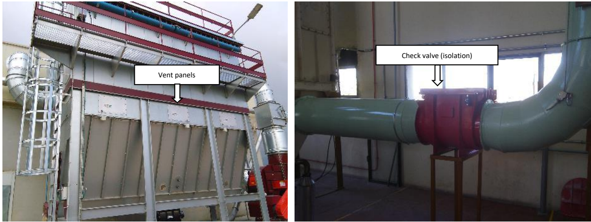
Fig. 4. Protection systems in baghouses
