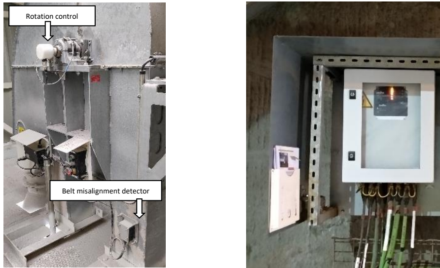
Fig. 3 Elevator ignition source control system (Spyline ADIX)
