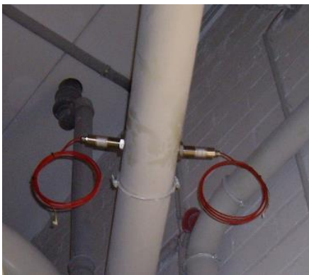
Fig. 2 Spark detection and extinguishing system (source: T&B Electronic GmbH).
